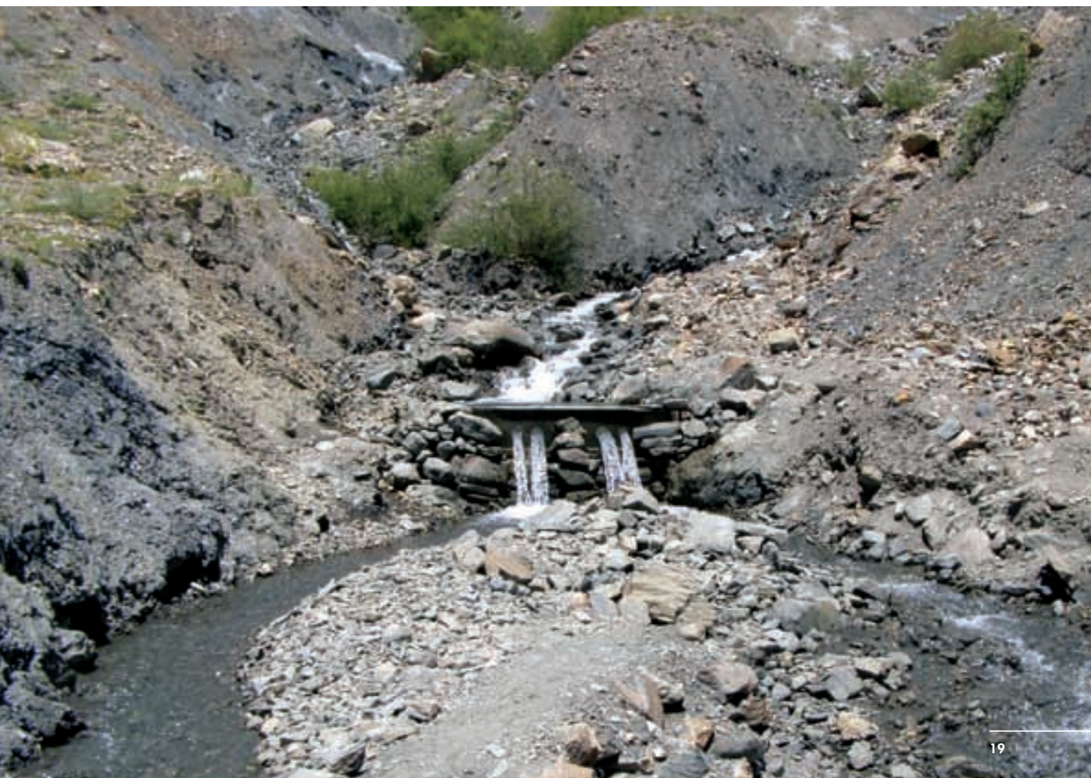
Traditional water distribution and control structure (nirwalu) in Mulkhow for dividing water in equal portions for two downstream users
