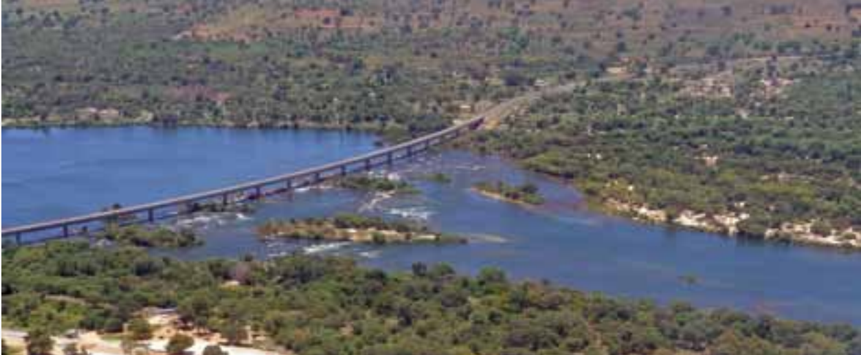
Bridge in the Southern African Development Community (SADC)
